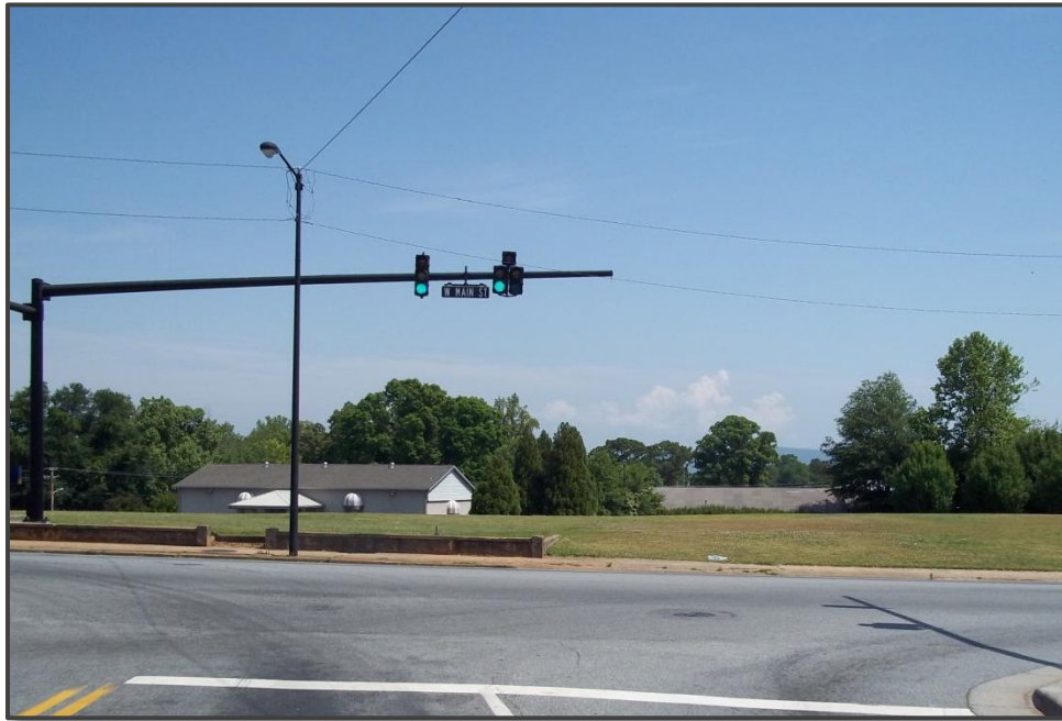
Figure 12: Example Building on West Main Street at Church Street
