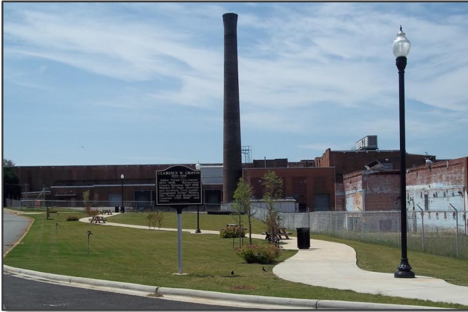
Figure 9: Mill Street Enhancement Project
