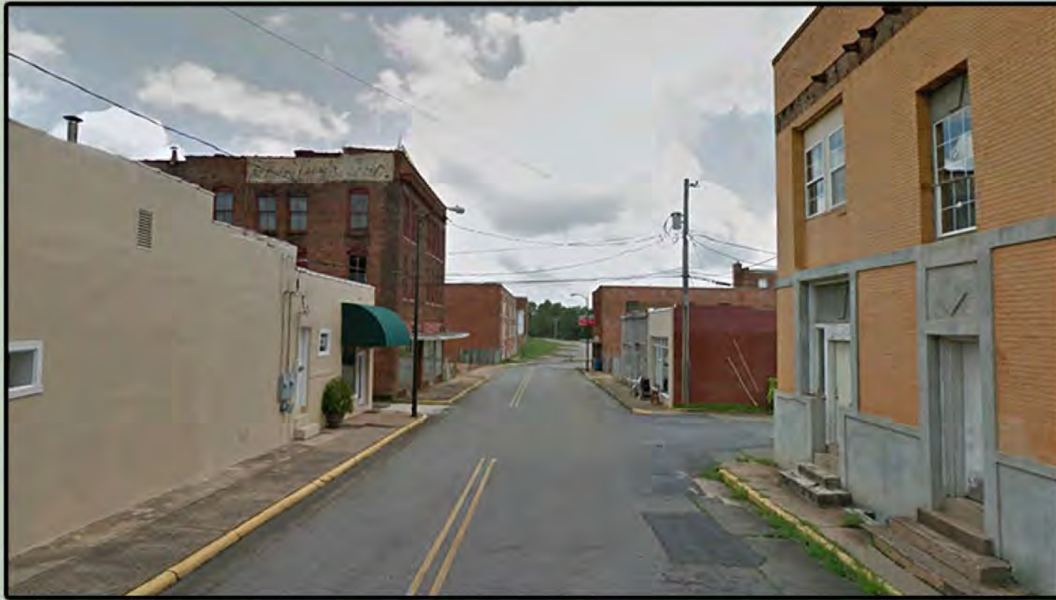
DEPOT STREET & EAST MAIN STREET BEFORE
