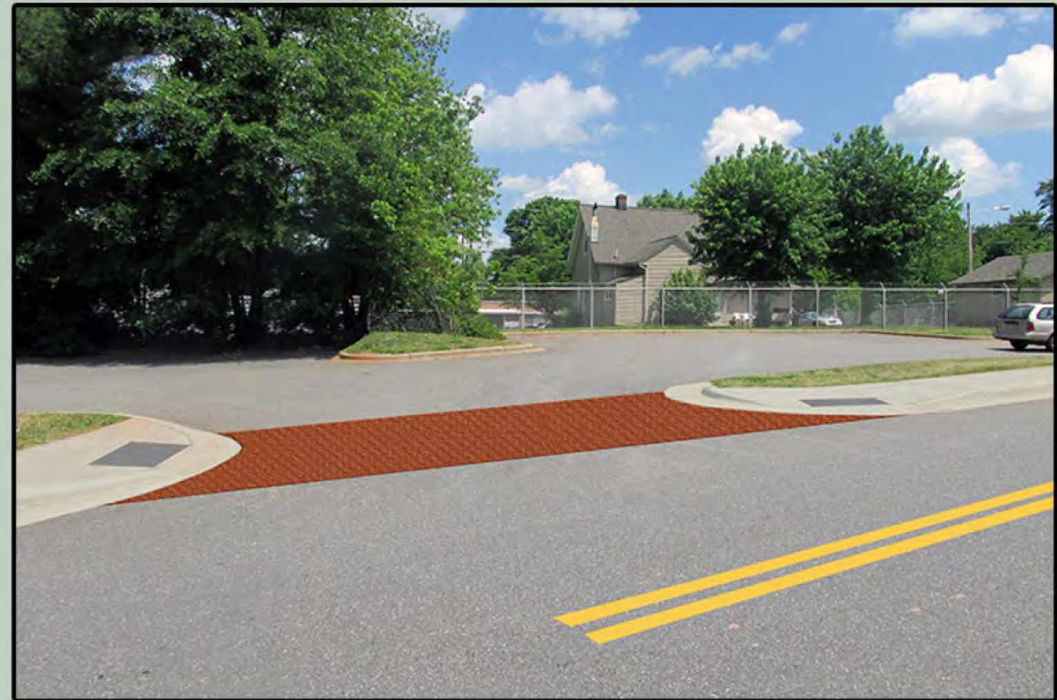
MILL STREET CURB CUTS AFTER
