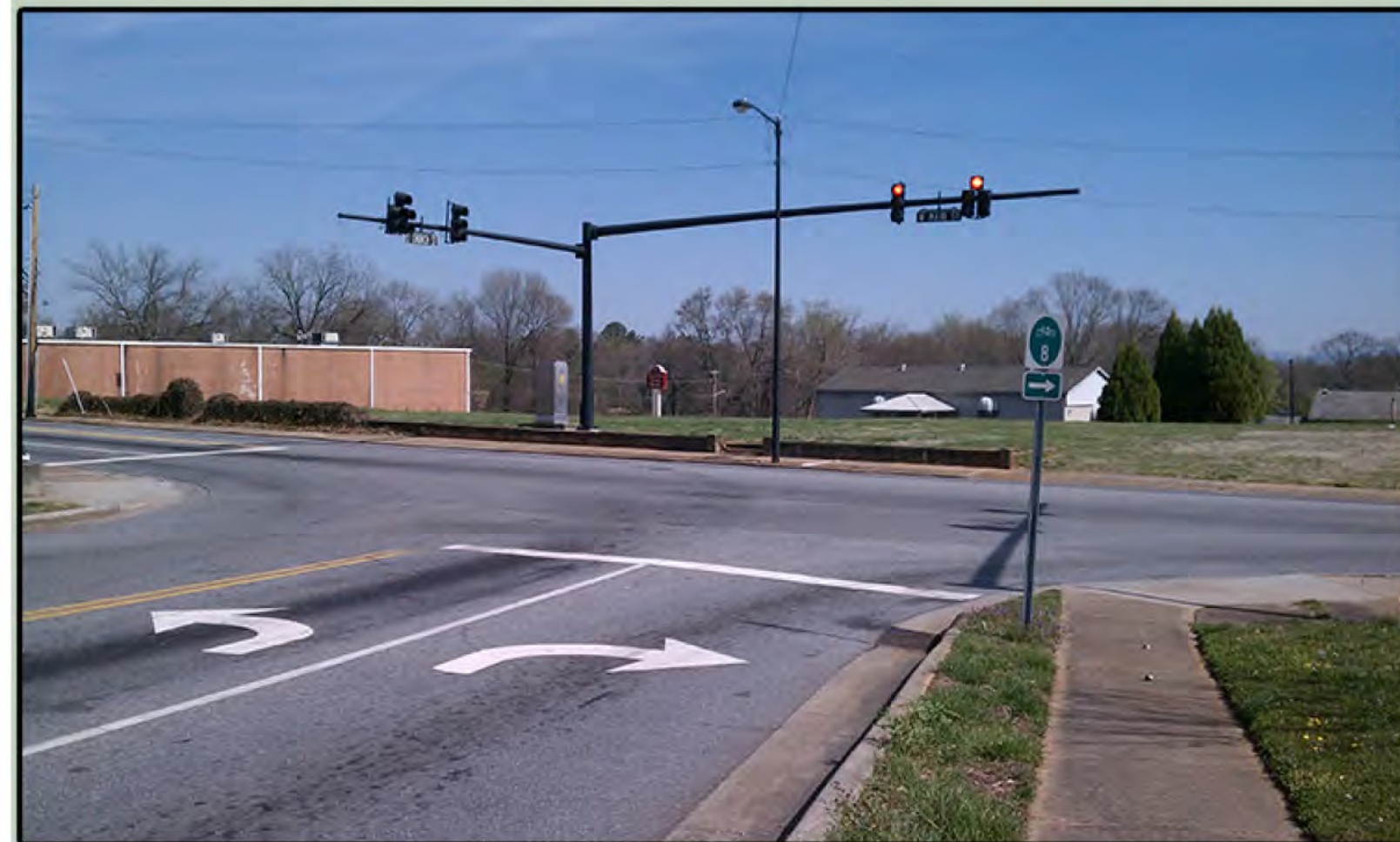
WEST MAIN STREET AND CHURCH STREET INTERSECTION BEFORE
