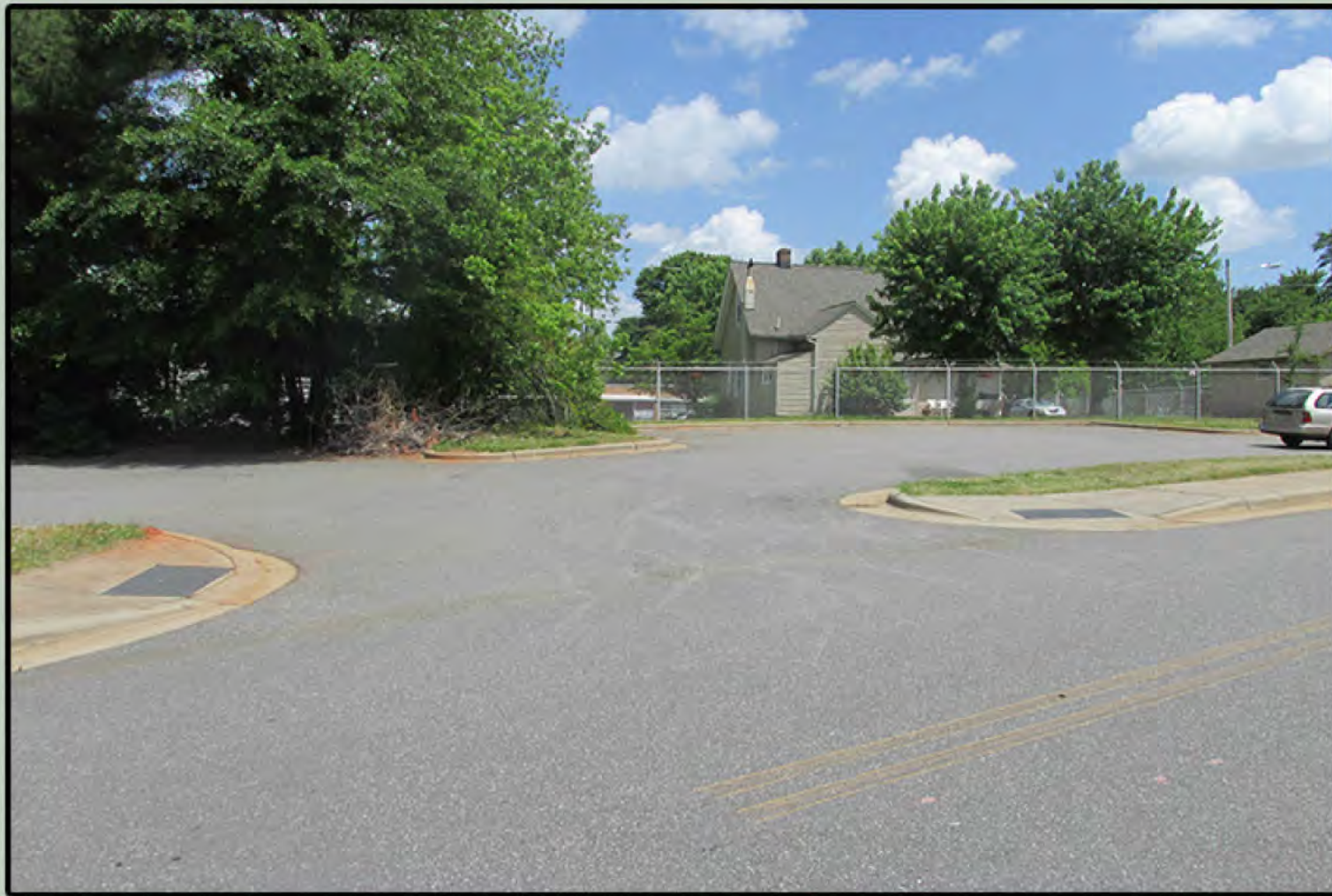
MILL STREET CURB CUTS BEFORE
