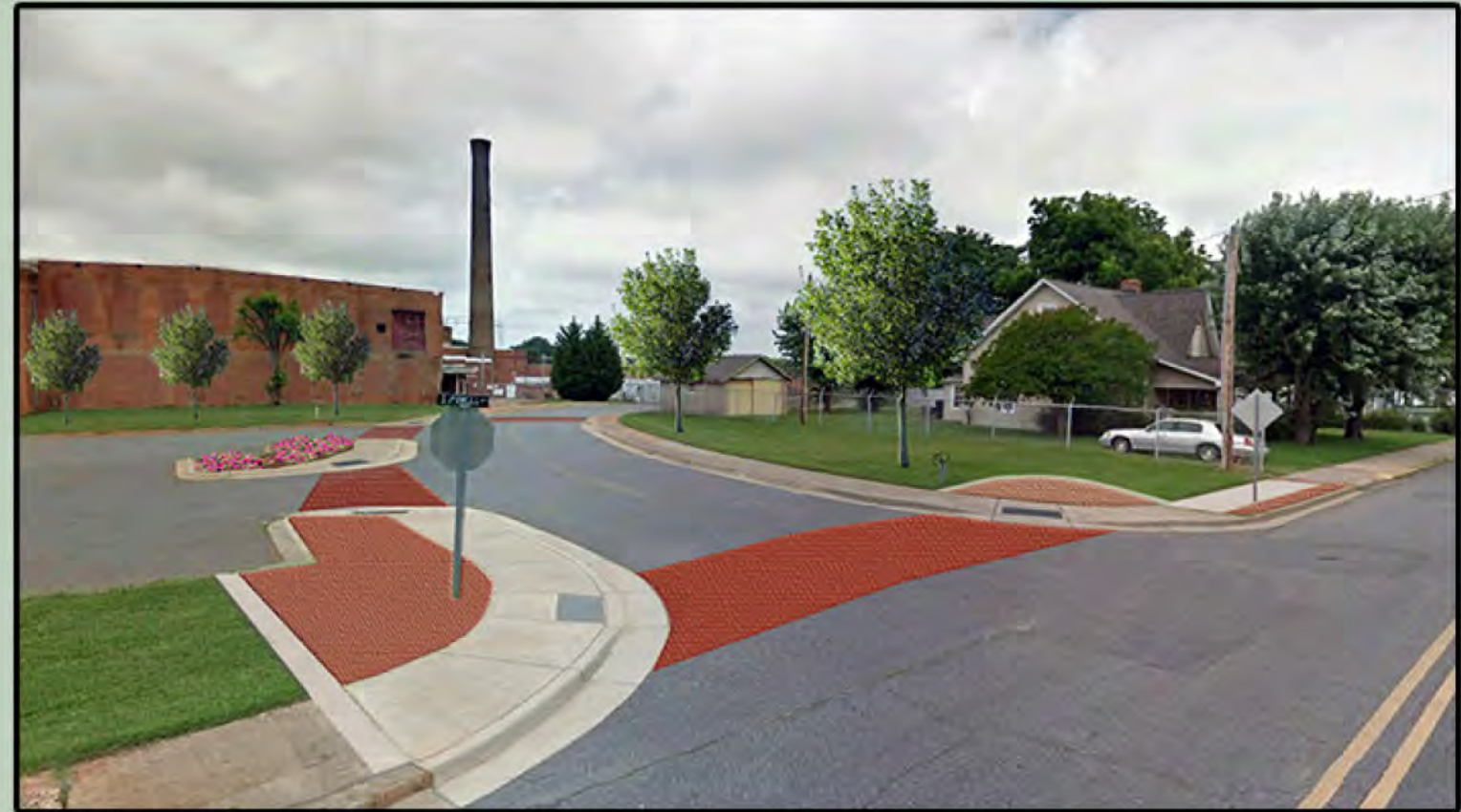
POWELL STREET & MILL STREET AFTER
